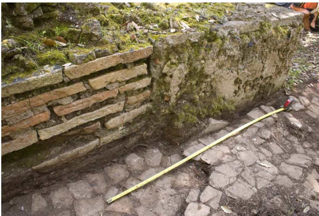
Fig. 38 Vicus A21 junction of floor with south face of plunge pool A22
