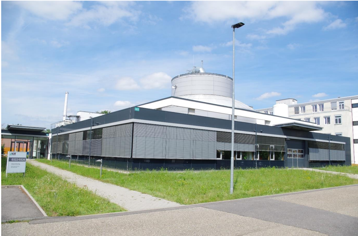
The IMK's department for Atmospheric Aerosol Research, home to the cloud chamber and the AWiCiT experiments. The dome and cylinder that can be seen protruding from the middle of the building house the upper heights of the cloud chamber.
