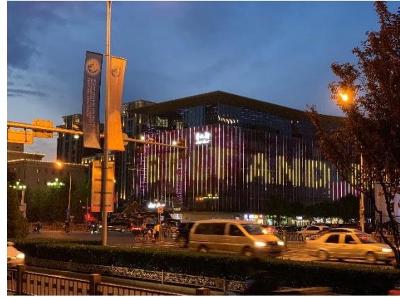
Animation Display (Belt and Road) on the curtain wall of the Silk Street Market
